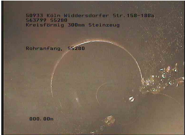
1, 00:00:00, 0.00m Rohranfang, S5280
