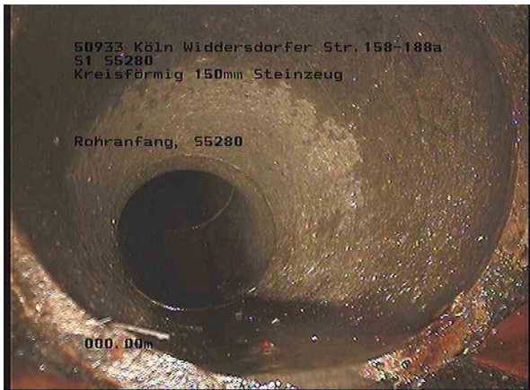
1, 00:00:00, 0.00m Rohranfang, S5280
