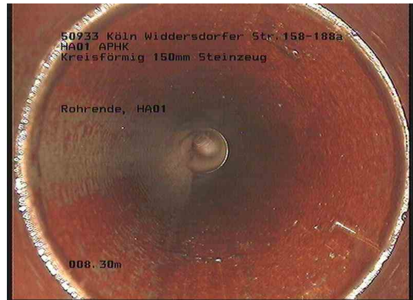
2, 00:01:32, 8.30m Rohrende, HA01 / SK
