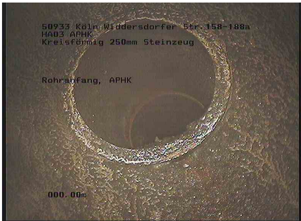
1, 00:00:00, 0.00m Rohranfang, APHK
