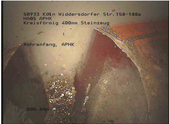
1, 00:00:00, 0.00m Rohranfang, APHK
