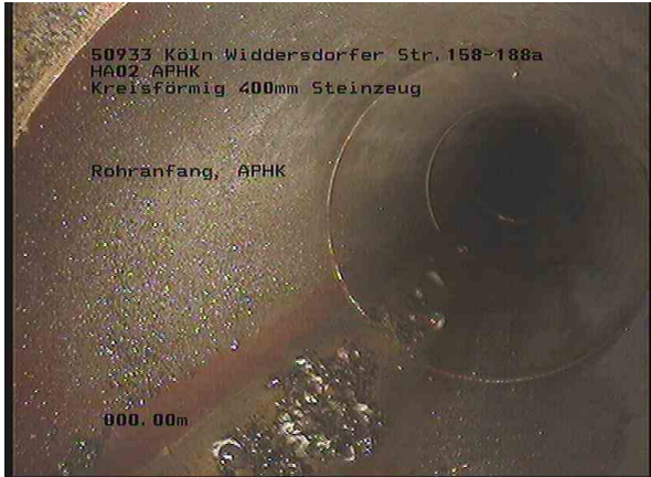
1, 00:00:00, 0.00m Rohranfang, APHK
