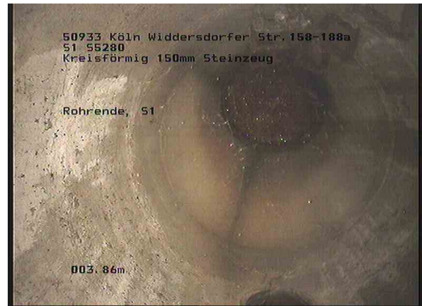
2, 00:01:06, 3.86m Rohrende, S1
