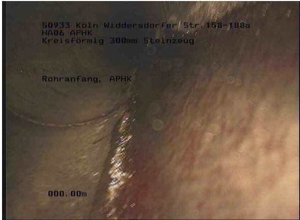
1, 00:00:00, 0.00m Rohranfang, APHK
