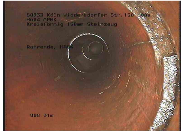
2, 00:02:50, 8.31m Rohrende, HA04 / SK
