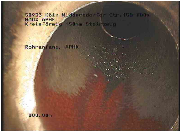
1, 00:00:00, 0.00m Rohranfang, APHK
