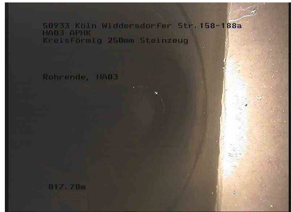
2, 00:02:39, 17.70m Rohrende, HA03
